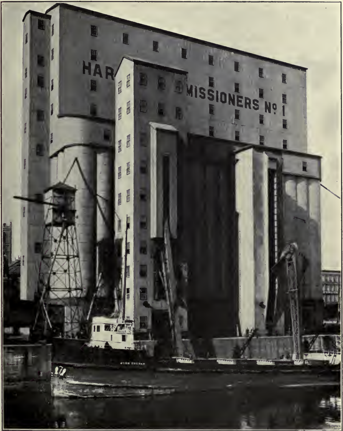
COMMISSIONERS ELEVATOR NO. 1, MONTREAL.
